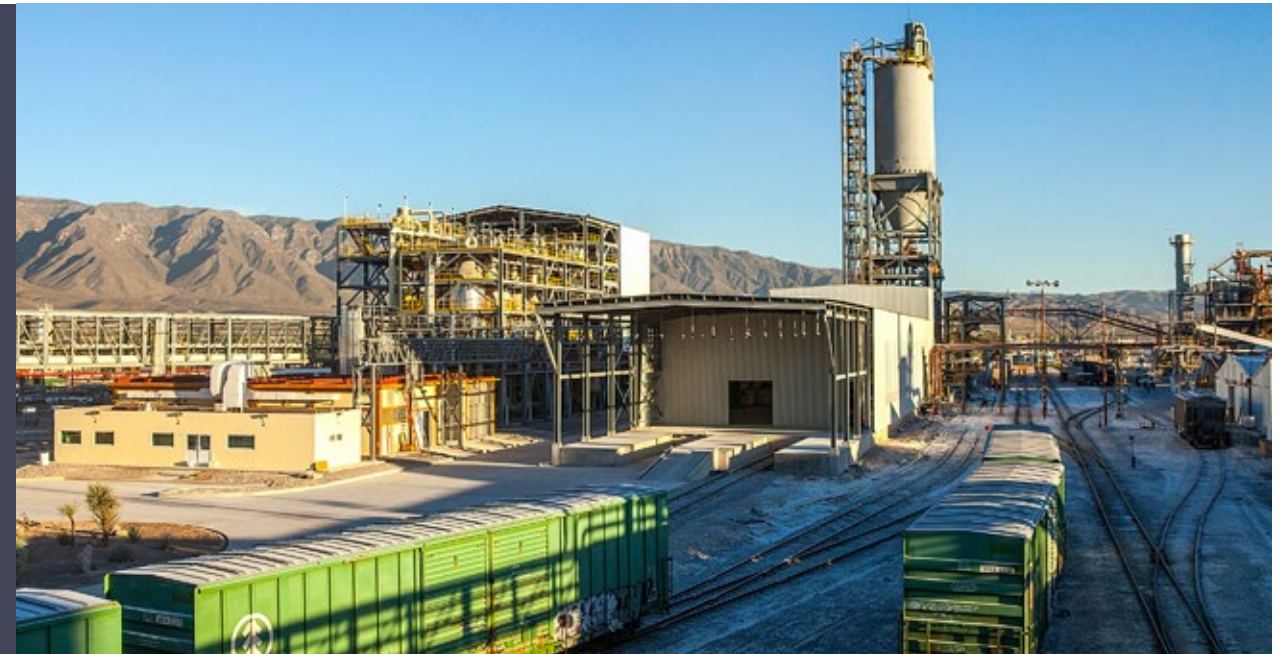
Transport yard at Química del Rey
