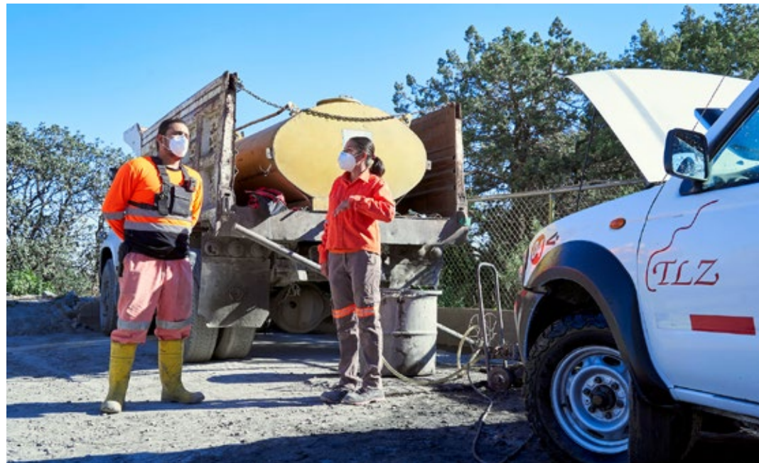
Contractor at the Sabinas unit
