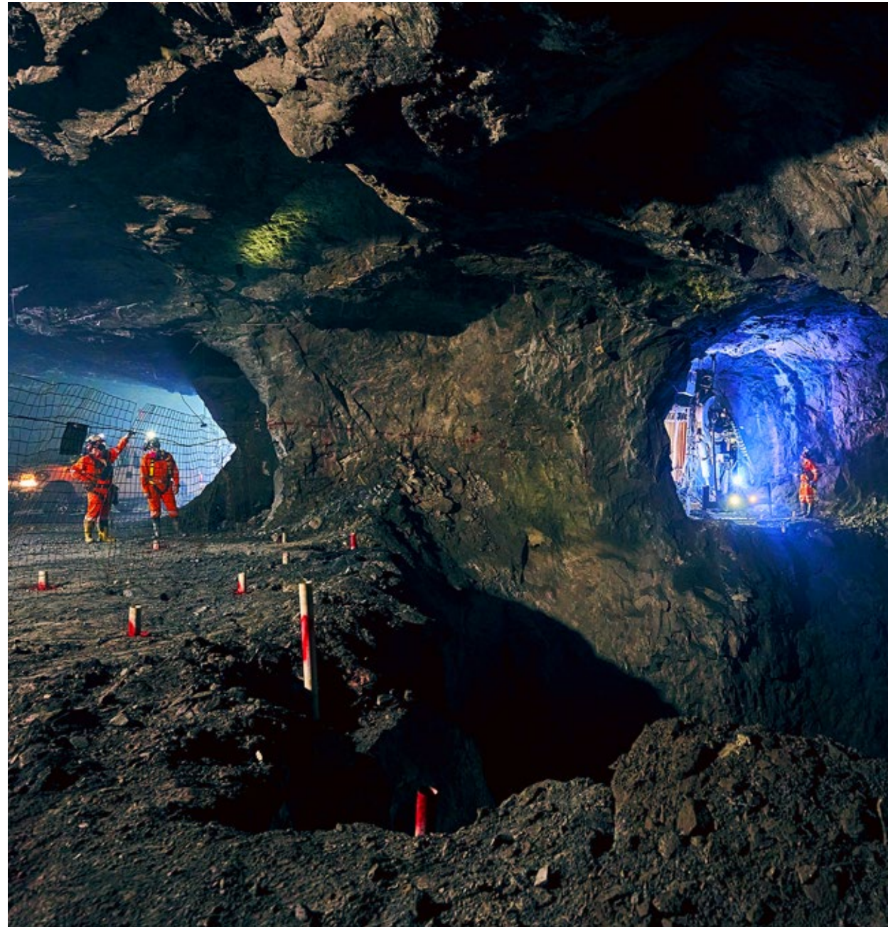
Simba drilling equipment inside Sabinas unit
