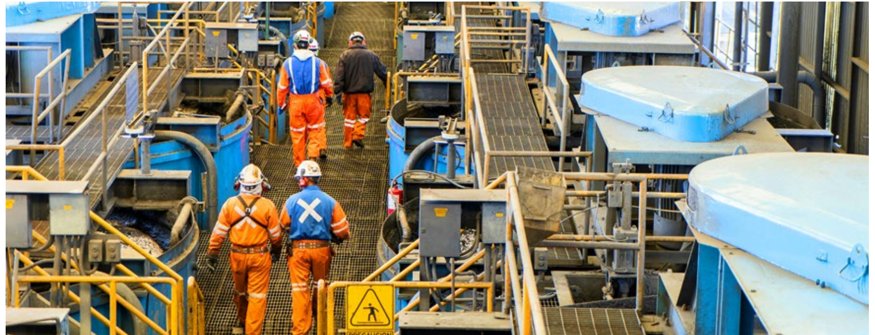
Flotation area at Madero unit
