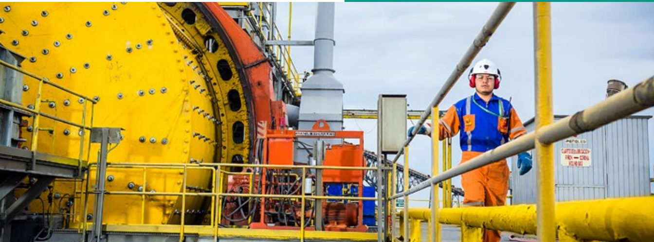
Grinding unit, Madero plant
