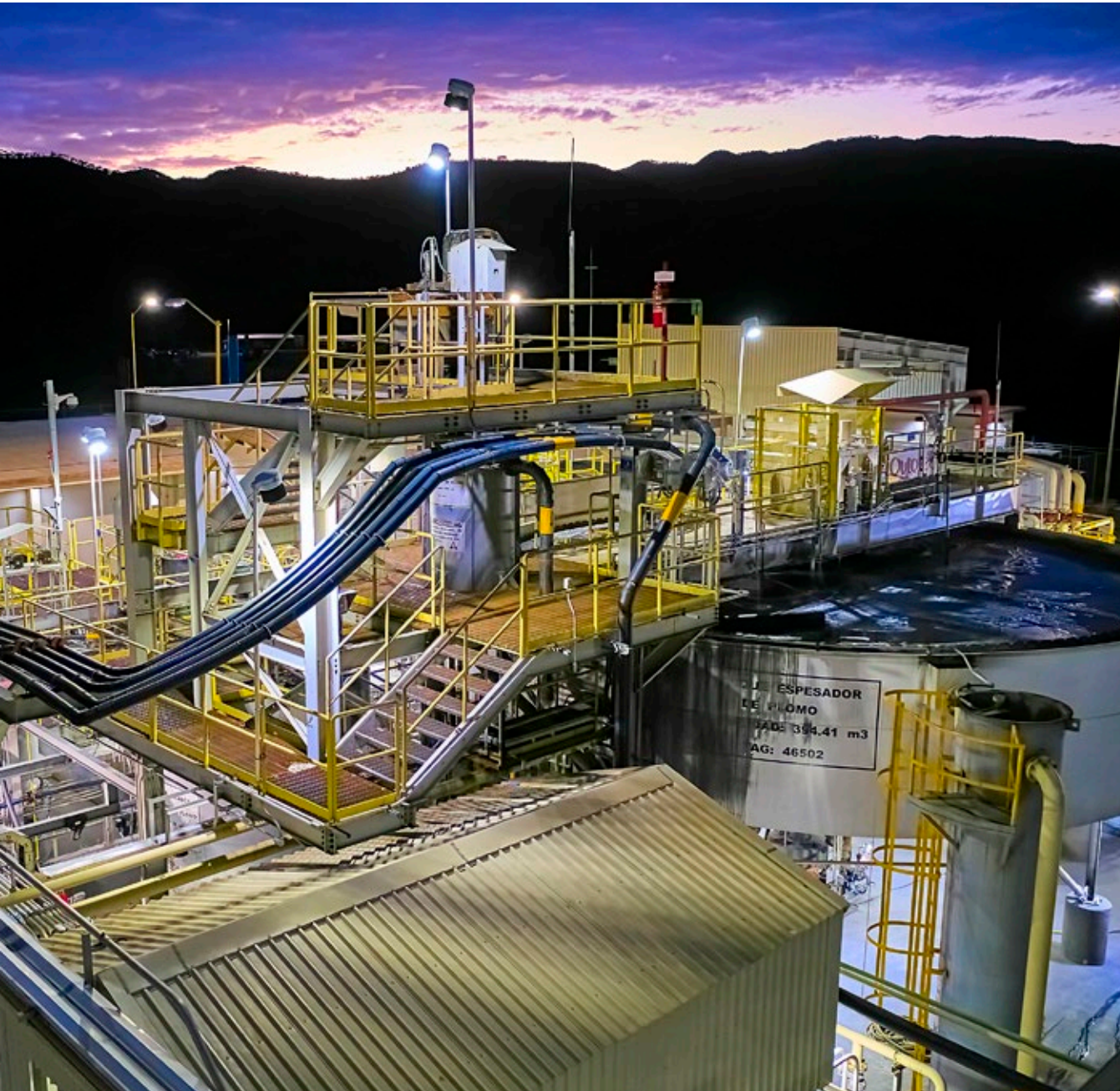
Aerial view at sunset, Capela unit
