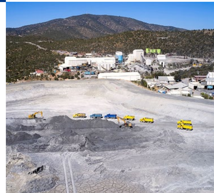
Conditioning of tailings dam at Sabinas unit
